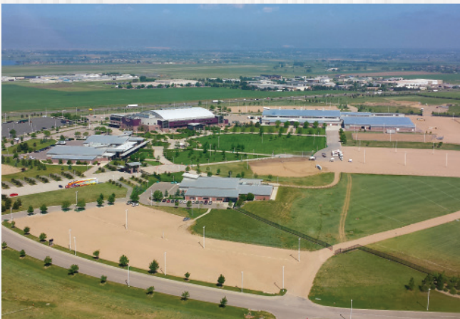
375,000 Square Feet of Event Space
